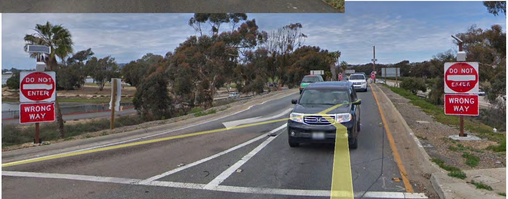
TraffiCalm System at Sea World Drive & SB I-5 in District 11
