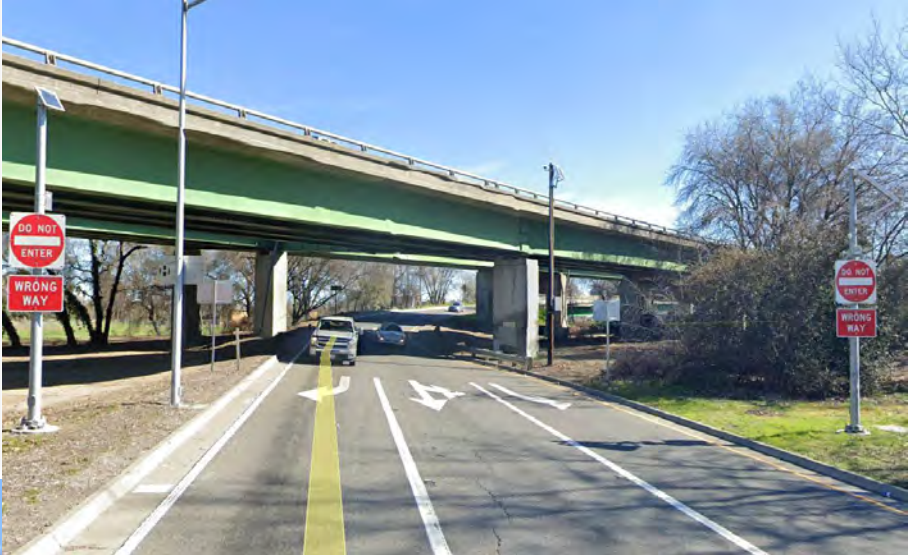
TAPCO System at Jefferson Blvd & WB US 50 in District 3
