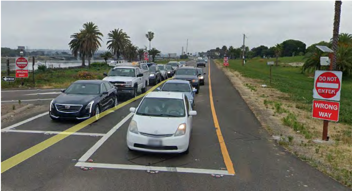
TraffiCalm System at Sunset Cliffs Blvd & WB I-8 in District 11
